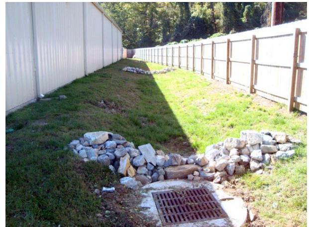
Check dams in a grass channel slow runoff. They can be made of rocks, as above, or timbers, concrete, or other suitable material.
