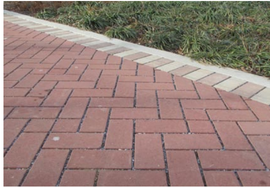
Upper left: Pervious pavers installed at Elmwood Park.
