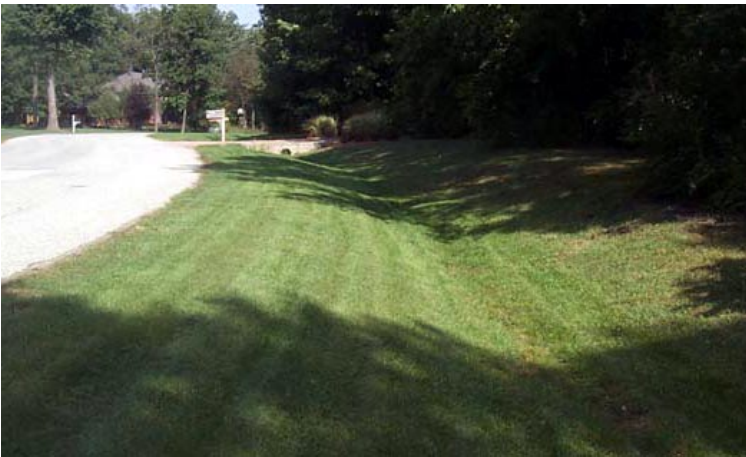
A grass channel along a residential street. Photo by the Natural Resources Conservation Service
