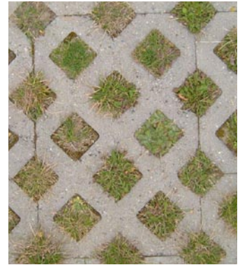
Upper left: Pervious pavers installed at Elmwood Park.
