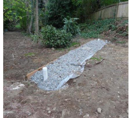
This backyard infiltration trench (under construction) will receive runoff from downspouts, as well as surface runoff. (photo by Ian Maddox)
